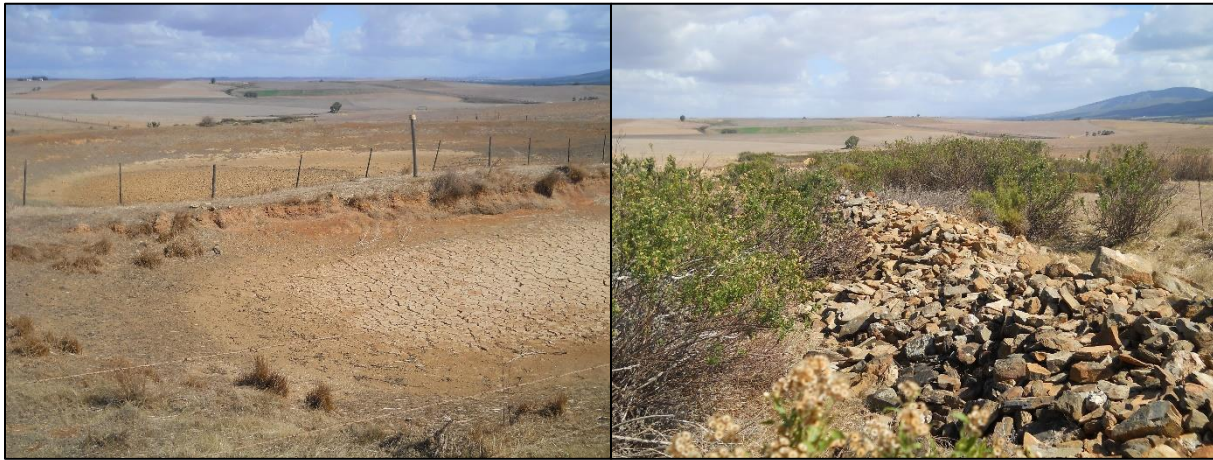
Figure 8: Impoundments within the upper reach of the wetland (left) and rocks stockpiled within the wetland (right).
