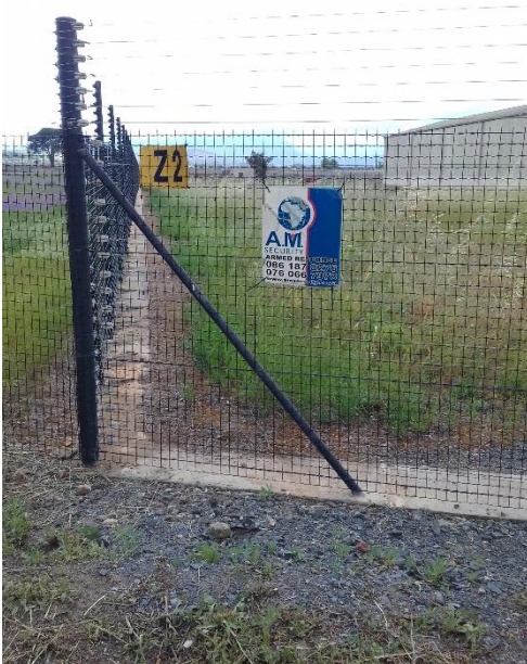
Photo 3: The proposed site has no natural vegetation and is located on an undeveloped part of the property. Photo taken from Vlottenburg Road.
