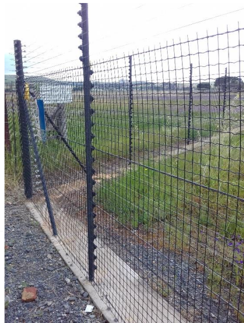
Photo 4: The proposed site is surrounded by an electric fence.
