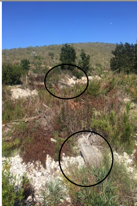
Figure 15 indicating the broken weir
