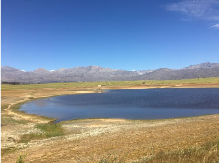
Figure 5: Photo taken on the eastern part of the dam wall facing south
