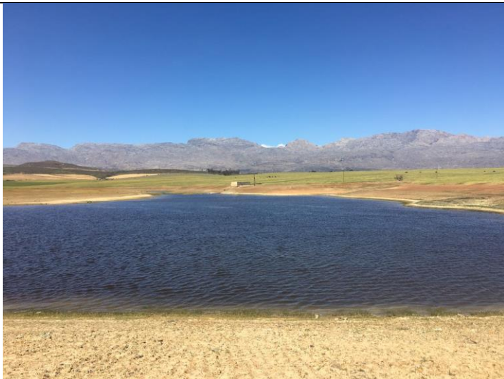
Figure 3: Photo taken standing in the middle dam wall facing south
