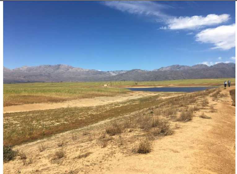
Figure 6: Photo taken from the far eastern part of the dam wall looking west towards to dam
