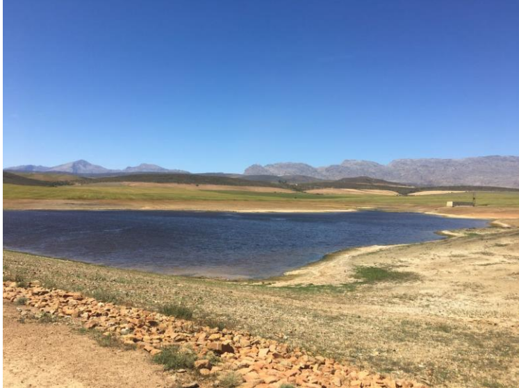
Figure 1: Photo taken standing on the western part of the dam wall facing South East
