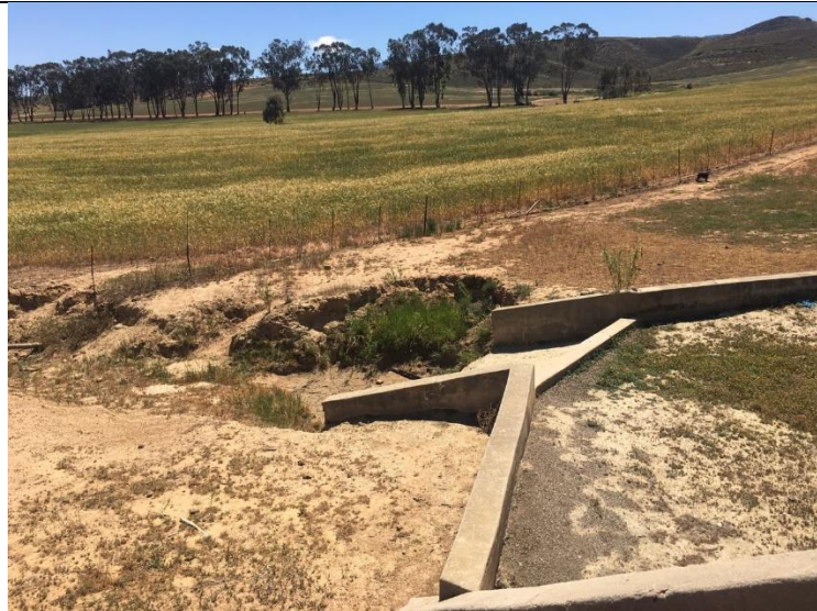
Figure 7: Spill way located on the north eastern part of the dam wall
