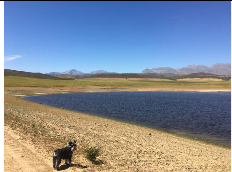
Figure 2: Photo taken standing in the middle of the dam wall facing south east
