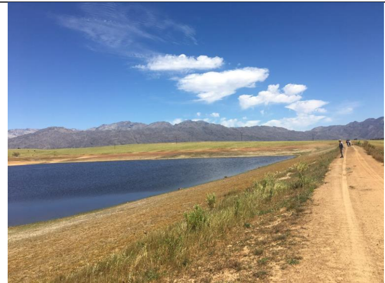
Figure 4: Photo taken standing on the eastern part of the dam wall facing West
