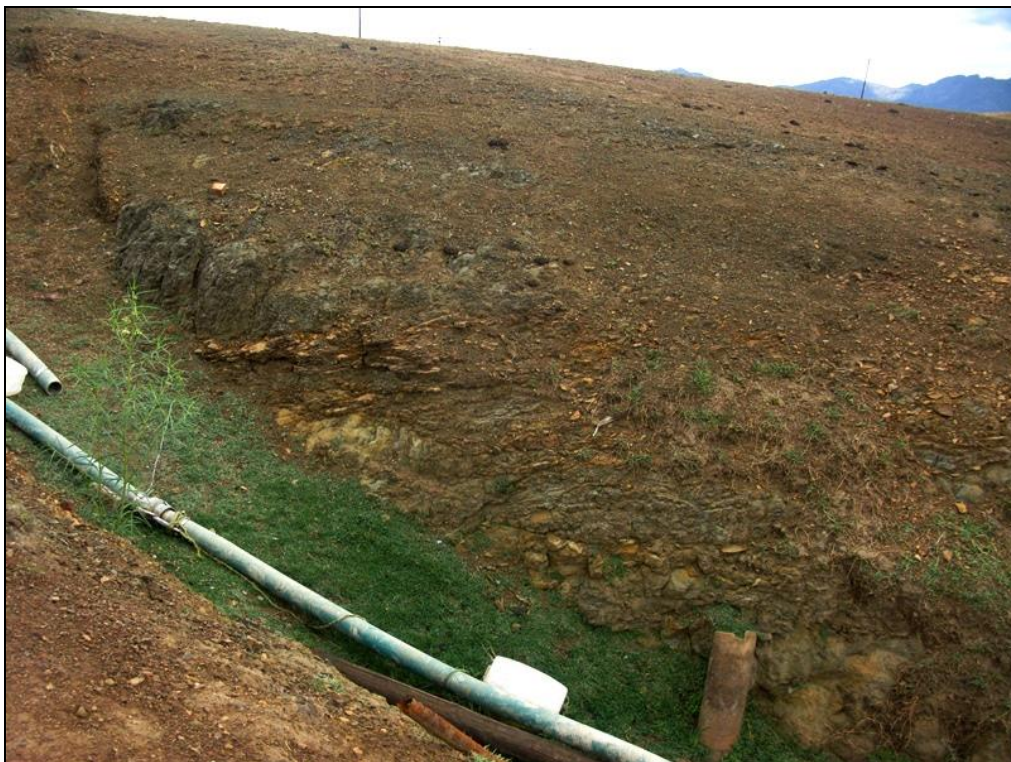
Figure 6: Highly fractured, faulted and weathered Voorstehoek Formation bedrocks exposed in a short pipeline trench on the southern edge of the existing dam.
