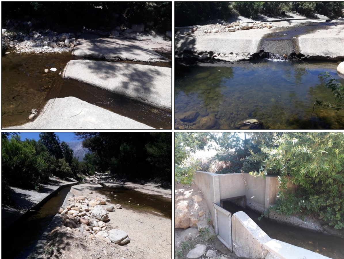
Figure 3: (Top left) existing diversion weir within the Wabooms River; (top right) downstream of the weir a pool has formed, water is abstracted from this pool for the Darling Brug Irrigation board; (bottom) diversion of water to a diversion chamber for the Wagenboom Irrigation Board.
