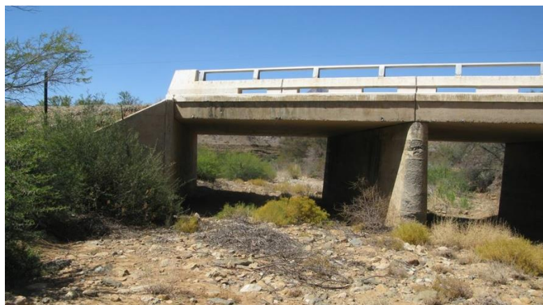
Figure 16: The bridge underneath the N14. The pipeline is proposed to be attached to this bridge.
