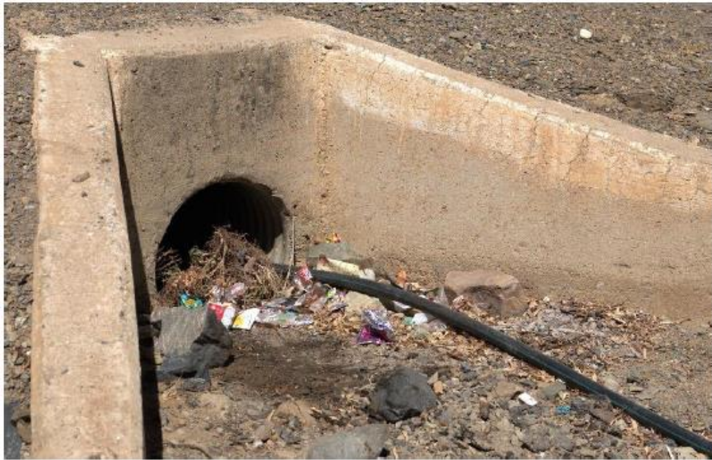
Figure 8: Culvert (Freshwater Report, WATSAN 2019)
