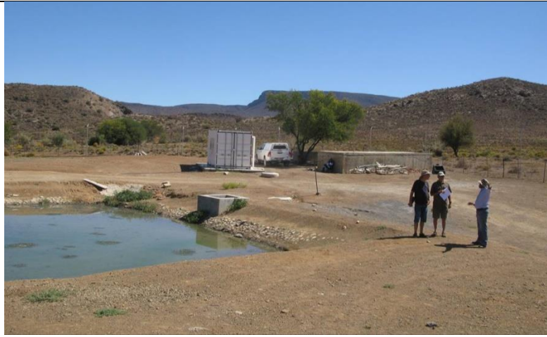
Figure 11: The existing WWTW looking from an easterly direction back towards the existing inlet structure of the WWTW. Again the absence of any natural vegetation within the fenced off treatment works footprint should be noted. A beautiful Vachellia karroo in the background next to the inlet works – clearly benefitting from the water on site (Botanical Impact Assessment, 2019).
