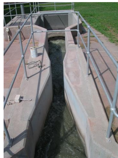
Figure 6: Parshall flume
