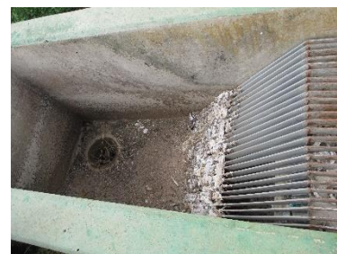
Figure 4: Hand -raked Screen
