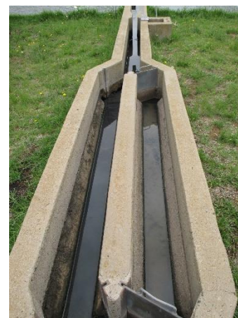
Figure 5: Dual Grit Channels
