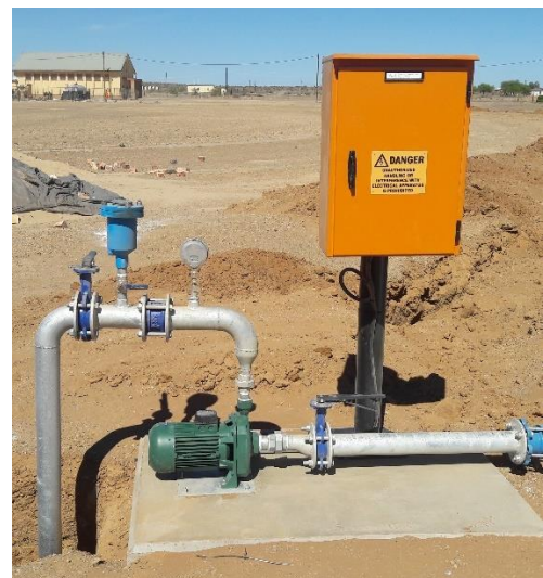
Figure 15: Irrigation Pump Station
