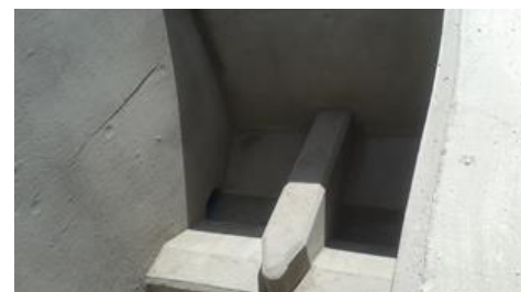
Figure 7 : Dividing Chamber or or Splitter Box
