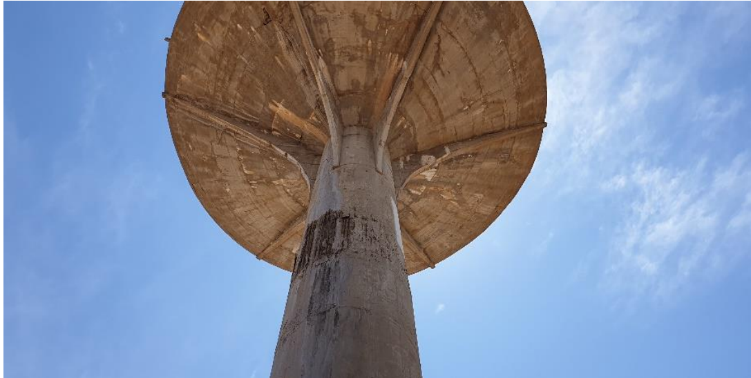
Figure 1: Exposed Reinforcement
