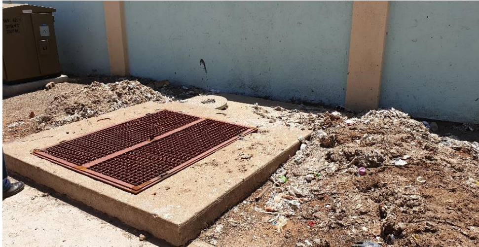
Figure 7: Lack of waste collection
