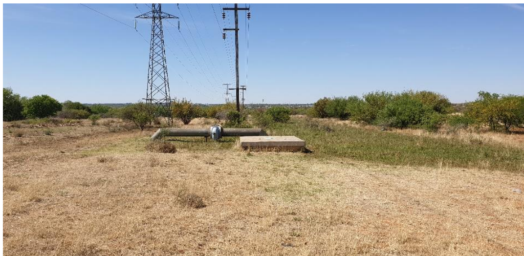
Figure 4: Main connection point with PRV chamber
