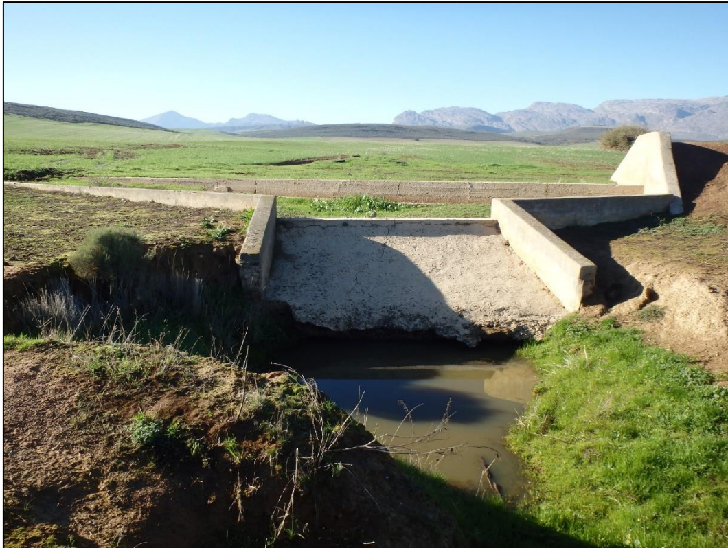
Figure 4: The existing spillway, located at the eastern end of the existing dam wall. Note the erosion and under-scouring at the spillway outlet.
