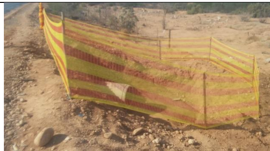
Figure 10 Footprint more clearly demarcated and disturbance rehabilitated
