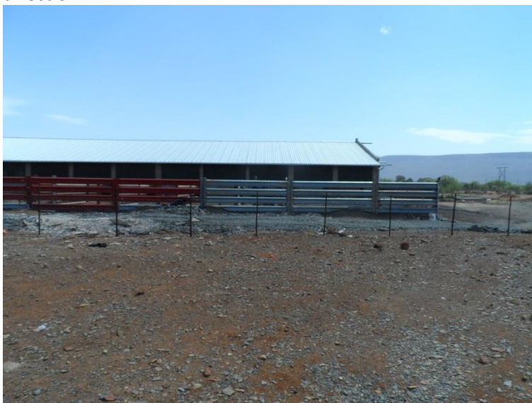
Picture 6: The pig pens, looking North at the south-eastern boundary of the property.
