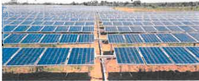
Figure 1: Single axis solar PV module tables raised 500mm above ground level
