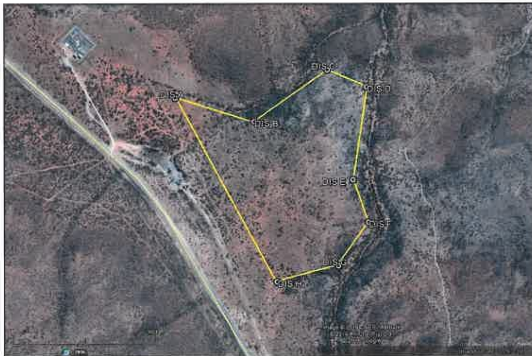
Fig. 13. Google earth© satellite image showing the revised study area for the Disselfontein Keren Solar Plant situated on the Remainder of Farm 77, Hopetown, close to the west bank of the Orange River and 23.5 km NW of Hopetown, Northern Cape (yellow polygon). Note that the previous field study (Almond 2012b) focused on the adjoining original study area situated close to the substation and quarry area to the northwest and west.
