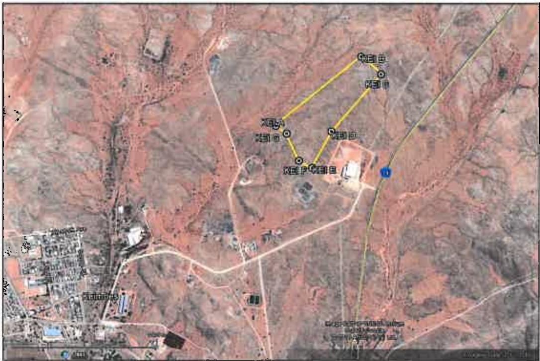
Fig. 2. Google earth© satellite image showing the study area for the Keren Keimoes solar farm on Erf 666 on the north-eastern outskirts of Keimoes and NW of the N14 trunk road, Northern Cape (yellow polygon).
