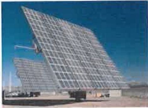
Figure 4: Typical CPV Unit
