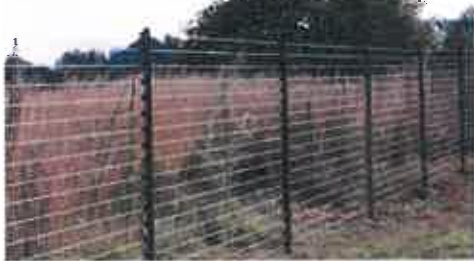
Figure 9: Typical electrical fence
