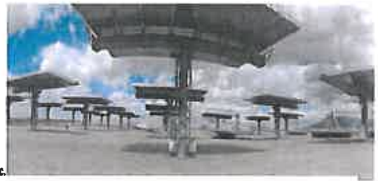
In stow: >20 m/h. > 10 sec. Out of stow: <25 m/h. >300 sec. Figure 4: Storm Stow position
