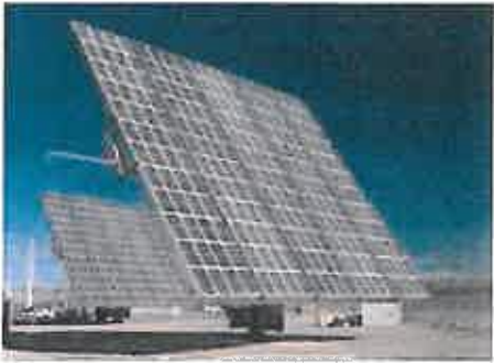
Figure 2: Typical CPV Unit
