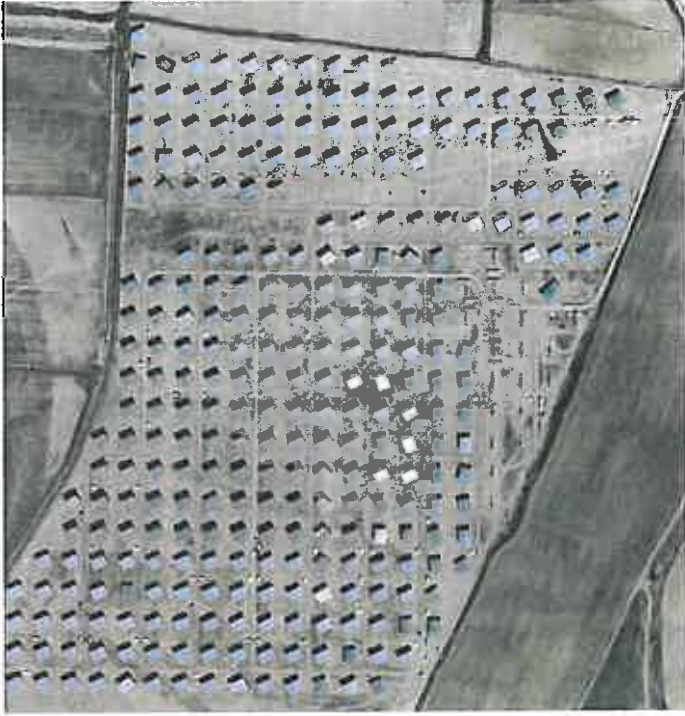
Figure 3: Typical Solar Farm layout
