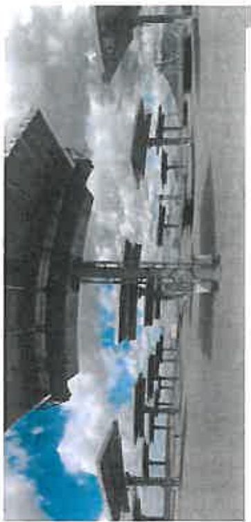
In stow: >28 mph, > 10 sec. Out of stow: <28 mph, >300 sec. Figure 6: Storm Stow position
