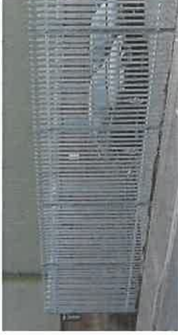
Figure 10: Typical galvanized palisade fence
