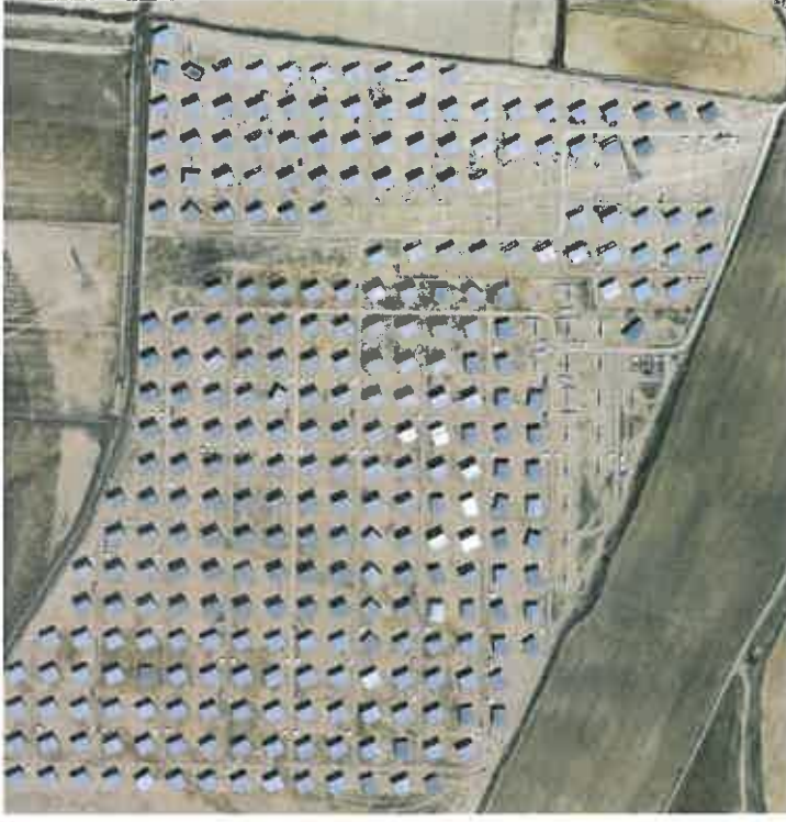
Figure 3: Typical Solar Farm layout
