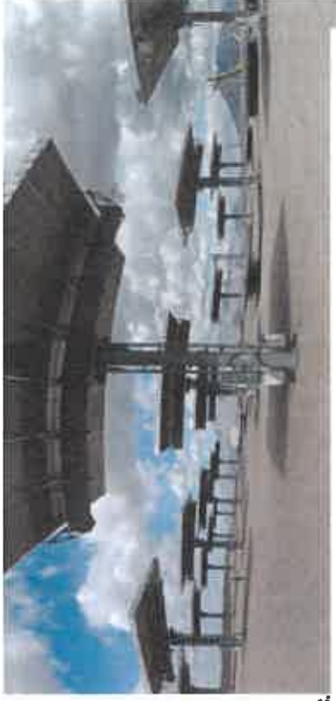
In stow: >28 mph, > 10 sec. Out of stow: <26 mph, >300 sec. Figure 6: Storm Stow position
