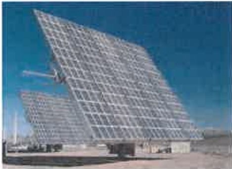
Figure 4: Typical CPV Unit
