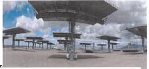
In stow: >28 mph, > 10 sec. Out of stow: <26 mph, >300 sec. Figure 6: Storm Stow position
