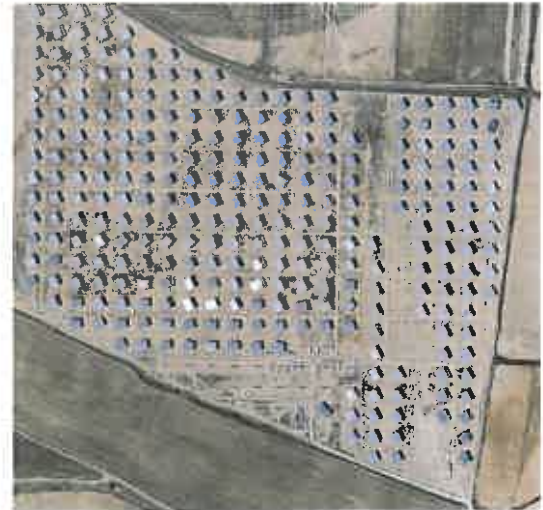
Figure 3: Typical Solar Farm layout
