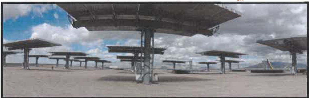
Photo 5: Typical layout of such a solar site (Image courtesy of Amonix, a leading designer of CPV technology)
