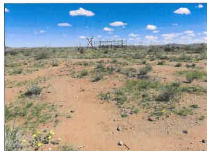
Figure 11. Site 0981. The Oasis substation is in the background
