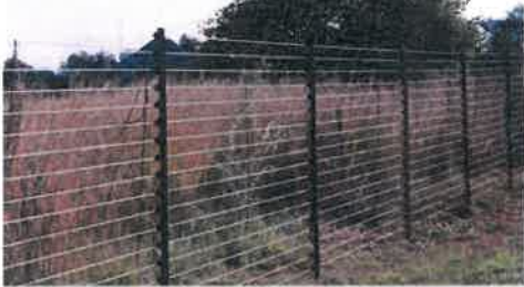
Figure 9: Typical electrical fence
