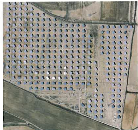
Figure 3: Typical Solar Farm layout
