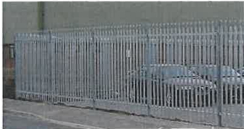
Figure 10: Typical galvanized palisade fence
