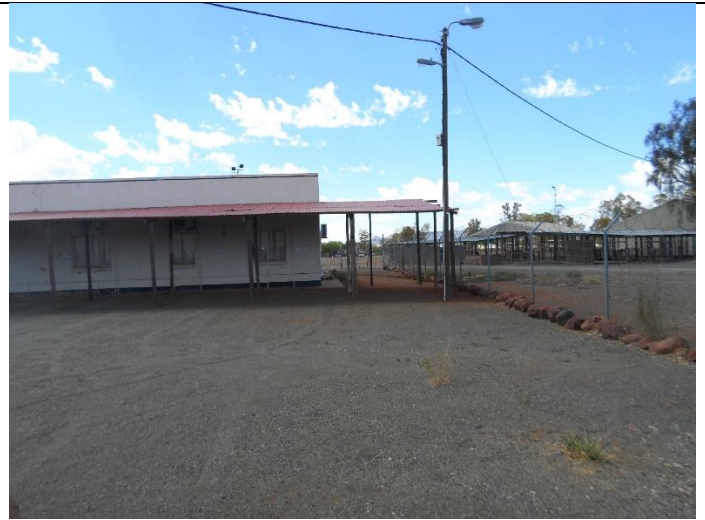
Figure 10: Looking towards the municipal building on the property as viewed from the site, looking in a southern direction.
