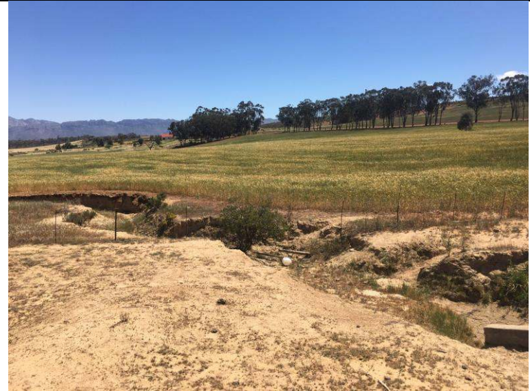
Figure 8: Highly degraded stream leaving Driefontein dam to the north of the dam
