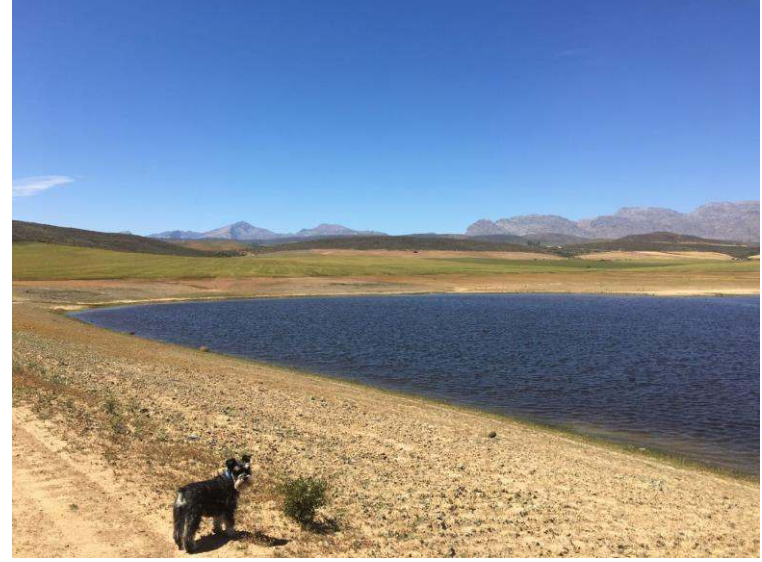
Figure 2: Photo taken standing in the middle of the dam wall facing south east
