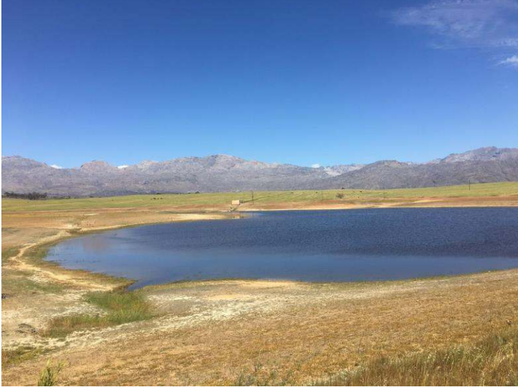
Figure 5: Photo taken on the eastern part of the dam wall facing south
