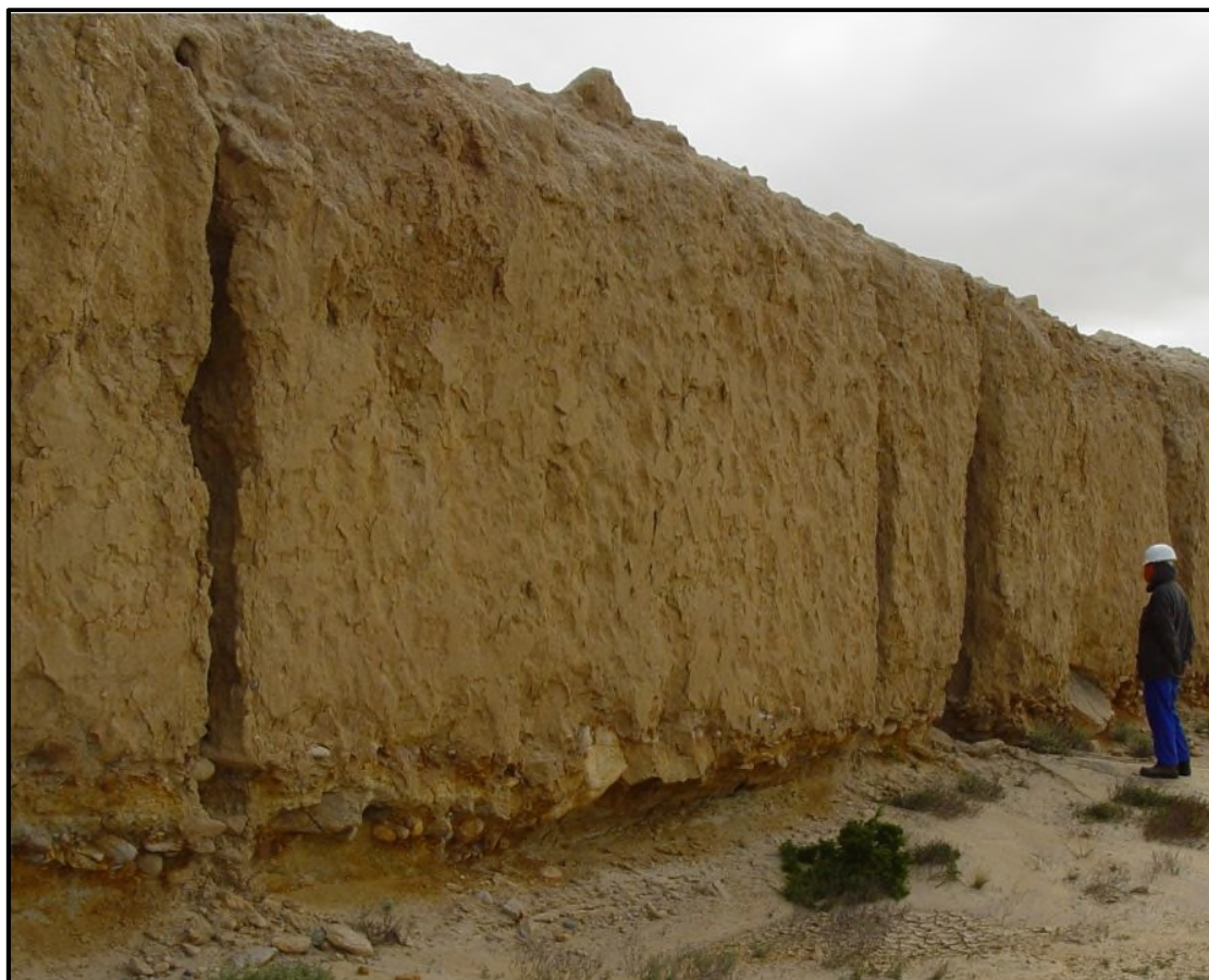
Figure 3. Typical section near Kleinzee. The capping calcrete has been stripped off.
