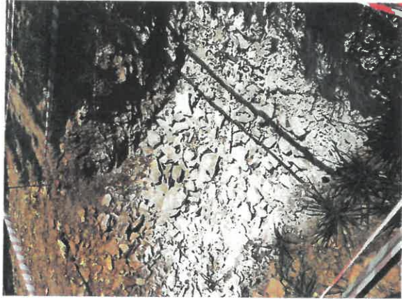
Figure 2: Lime in trench drains to prevent odour from wash water
