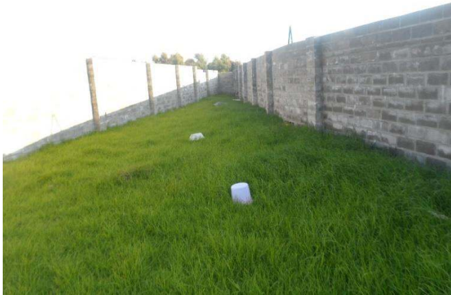
Figure 1: Area selected for the mast in the South – West corner of the property, RE Erf 5095 Broadlands
