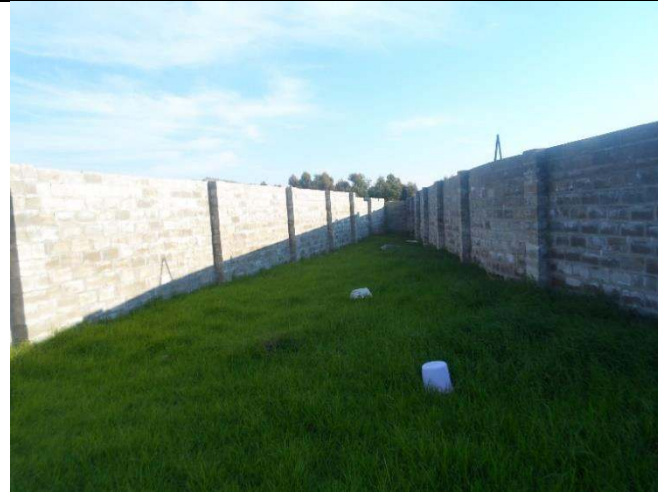
Figure 2: Area selected for the mast in the NE corner of the property, Erf 73 Klipheuwel
