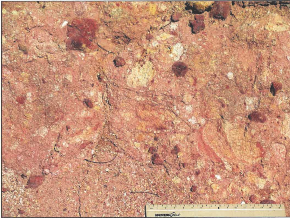
Figure 8. Close-up of pinkish, poorly sorted regolith with highly-weathered clasts of granite and reddish-brown ferruginous sandstone or ferricrete exposed in the upper part of the dam wall (Scale in cm). These deposits may be of ancient debris flow origin or were perhaps generated during dam wall construction.
