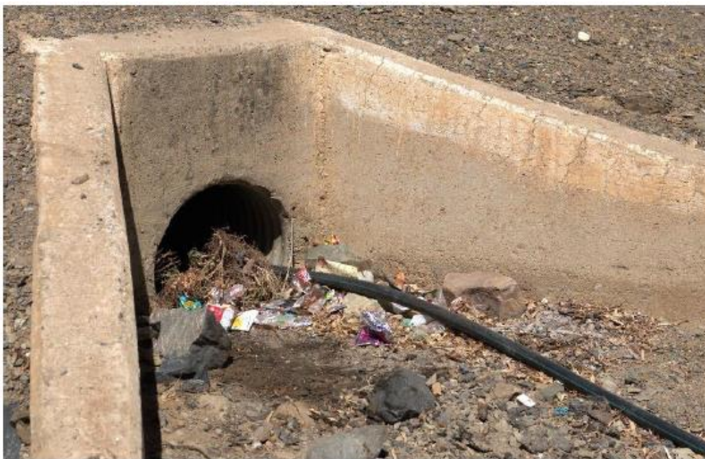
Figure 6: Culvert (Freshwater Report, WATSAN 2019)
