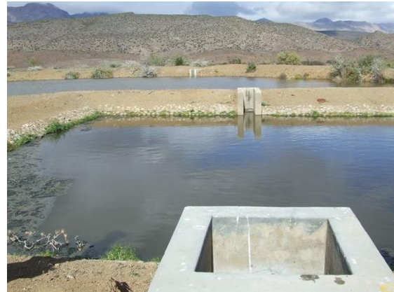
Figure 2: Existing Wastewater Pump Station and inlet to Anaerobic Pond
