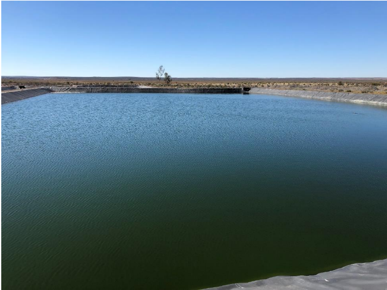
Typical Facultative Pond with full HDPE Lining, Brandvlei, Northern Cape
