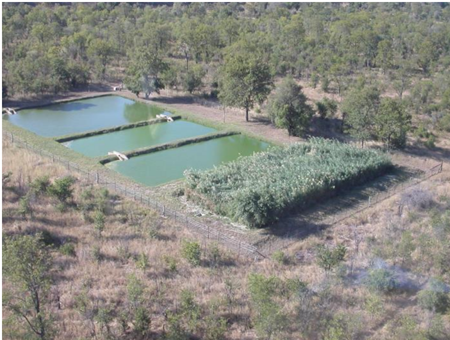
Figure 8: Example of an Oxidation Pond and Reedbed in the Kruger National Park
