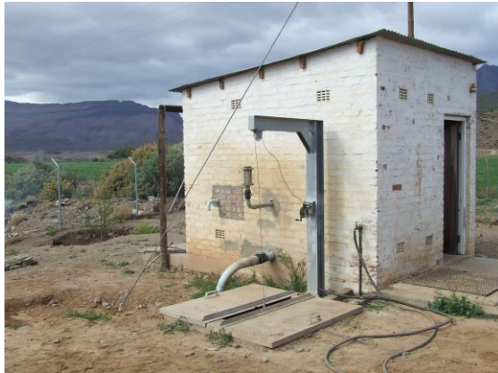
Figure 2: Existing Wastewater Pump Station and inlet to Anaerobic Pond
