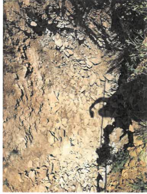
Figure 3: Lime in trench drains to prevent odour
