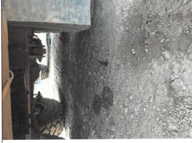
Figure 2: Oil spills from stationary water tank truck on site.
