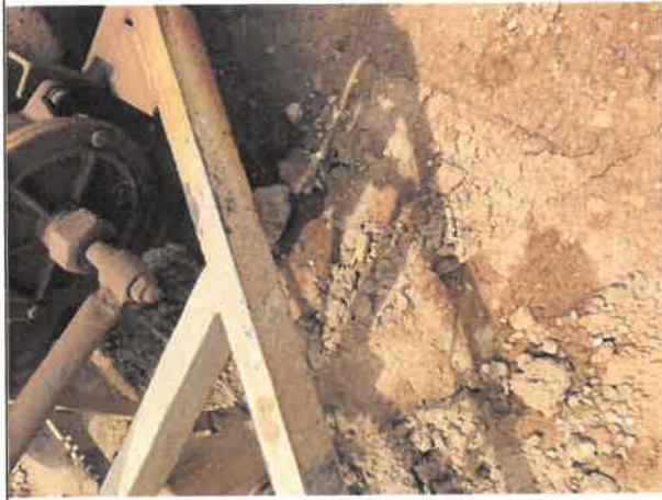
Figure 5: Previous Diesel spill under mobile refueler not cleaned up since last site visit (16 Nov) and still no drip tray placed.
