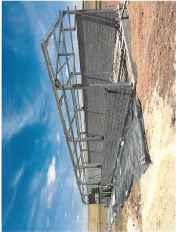
Figure 1: Dasberg Dam Pump house progress. Protective sheet placed for working with cement for protection
