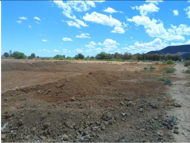
Figure 31: Trenches where condemned material was placed in and is covered in with soil after lime was added. Looking in a north-western direction.
