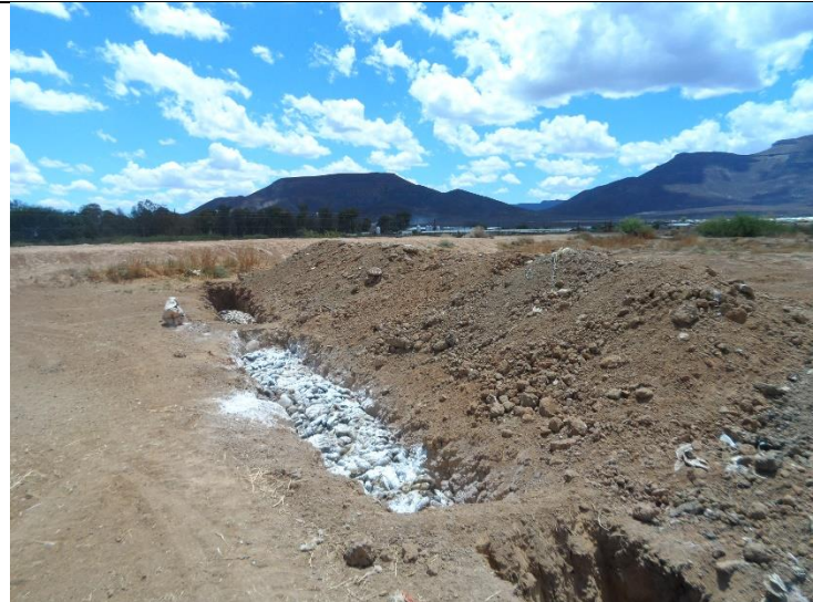
Figure 41: Condemned material placed in trenches; lime added and closed with soil. Looking in a north-western direction.
