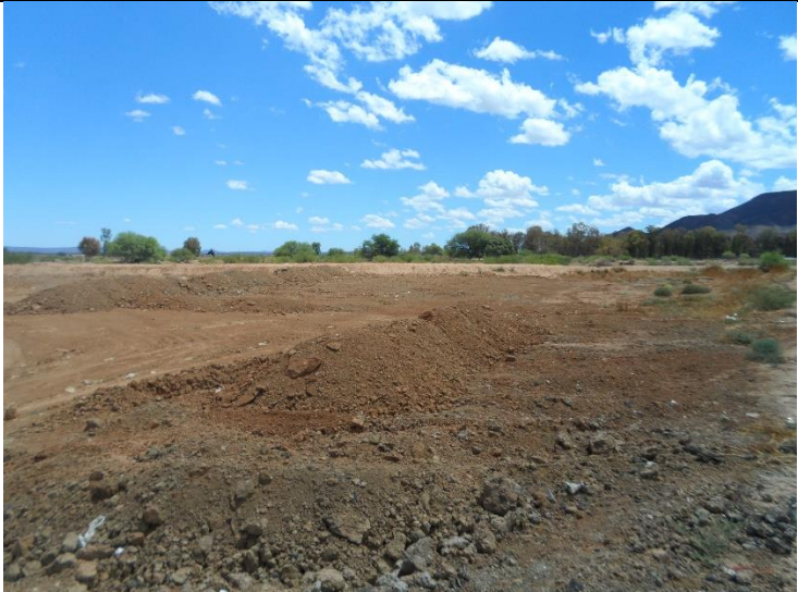
Figure 32: Trenches where condemned material was placed in and is covered with soil after lime was added. Looking in a western direction.
