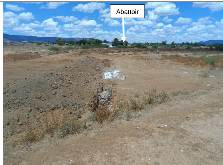
Figure 43: Condemned material placed in trenches; lime added and closed with soil. Looking in an eastern direction towards the abattoir.
