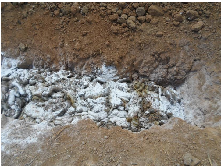
Figure 42: Condemned material placed in trenches; lime added and closed with soil.
