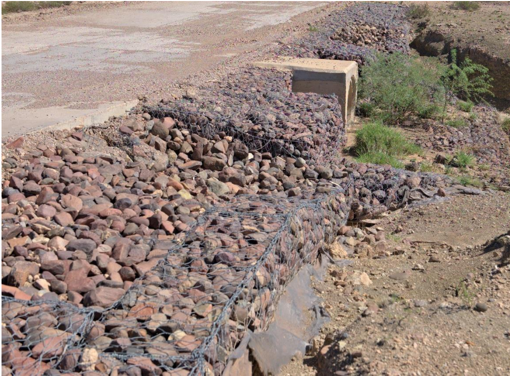
Figure 18 Partially collapsed gabions
