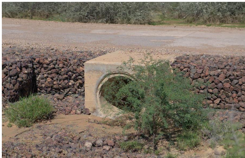
Figure 7 Storm water pipe under dirt road
