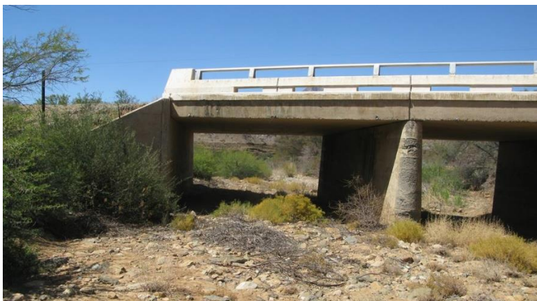
Photo 10: The bridge underneath the N14. The pipeline is proposed to be attached to this bridge.
