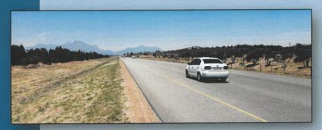
Stopping and Shoulder Sight Distances at the intersection will be more than adequate in both directions being on a stretch of the road that is very straight and flat.
