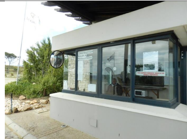
Figure 4: Close up of poster at La Grande Golf Estate
