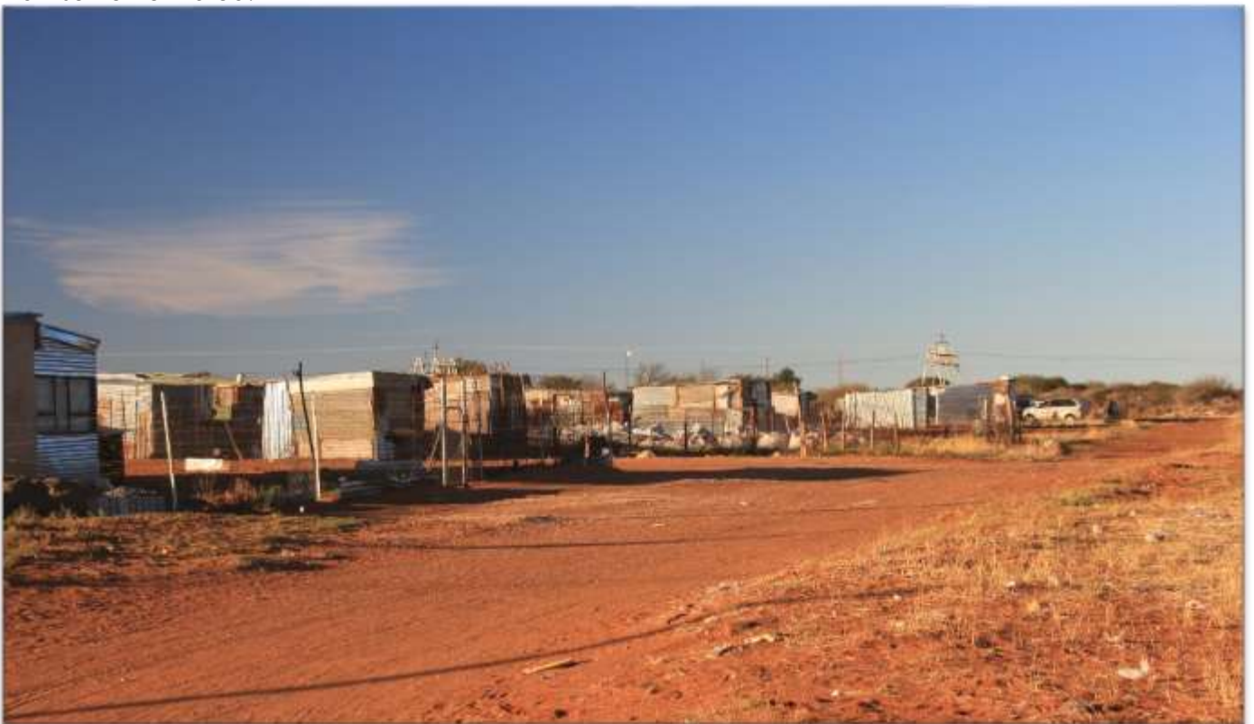
PHOTO 8: The image above shows some of the existing informal structures as are located on Remainder of the Farm Roodepan No. 70, Kimberley RD, as seen from a western direction, from the existing Ivory Park settlement area. At the back of the image the railway line is also visible. This railway was one of the important structuring elements during the layout planning and design phase of this project and was based on the specific inputs received from Transnet (see Annexure L).
