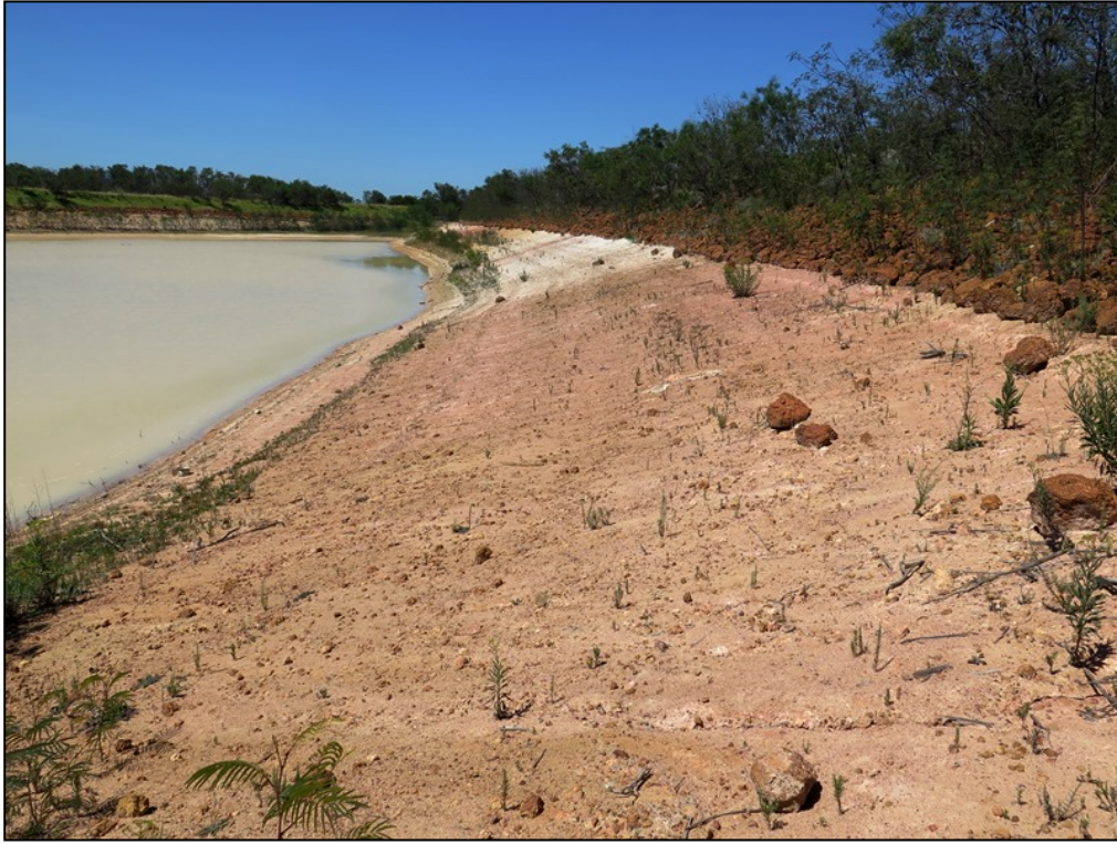
Figure 6. Deep excavation into pale cream to pinkish granitic saprolite and overlying weathered regolith along the margins of a large dam in the southern sector of Louw's Bos 502. The upper walls of the dam are armoured by locally-derived ferricrete blocks.
