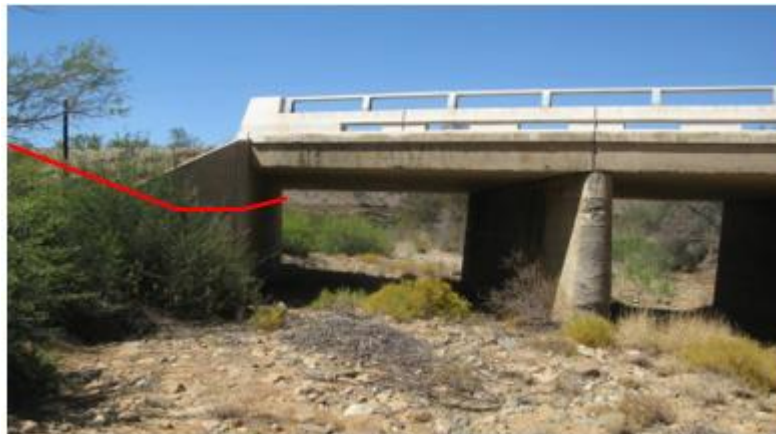
Figure 16: The bridge underneath the N12. The pipeline is proposed to be attached to this bridge.
