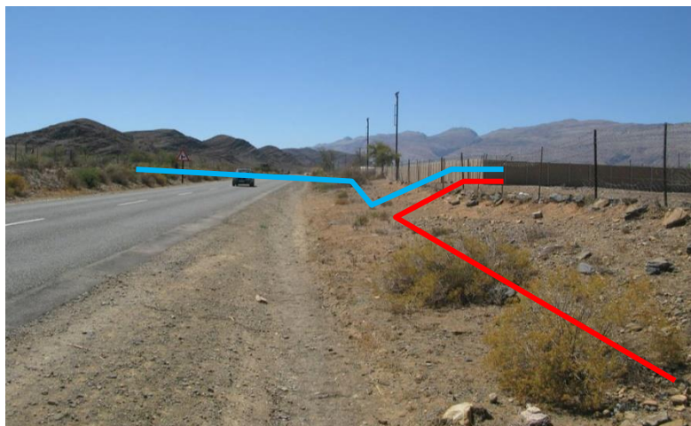
Photo 8: Showing the disturbed road reserve to the south of the N12. The blue line indicating the proposed preferred pipeline route, while the red line indicates the alternative route (not preferred).
