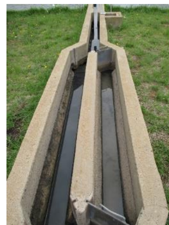
Figure 5: Dual Grit Channels
