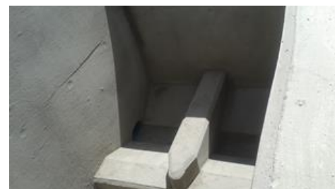
Figure 7 : Dividing Chamber or or Splitter Box
