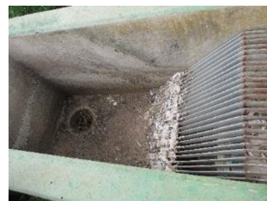
Figure 4: Hand -raked Screen
