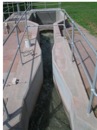
Figure 6: Parshall flume
