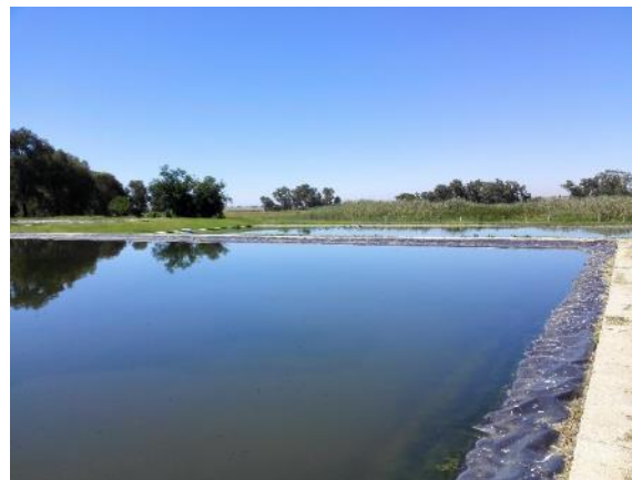
Figure 10: Typical Aerobic Pond
