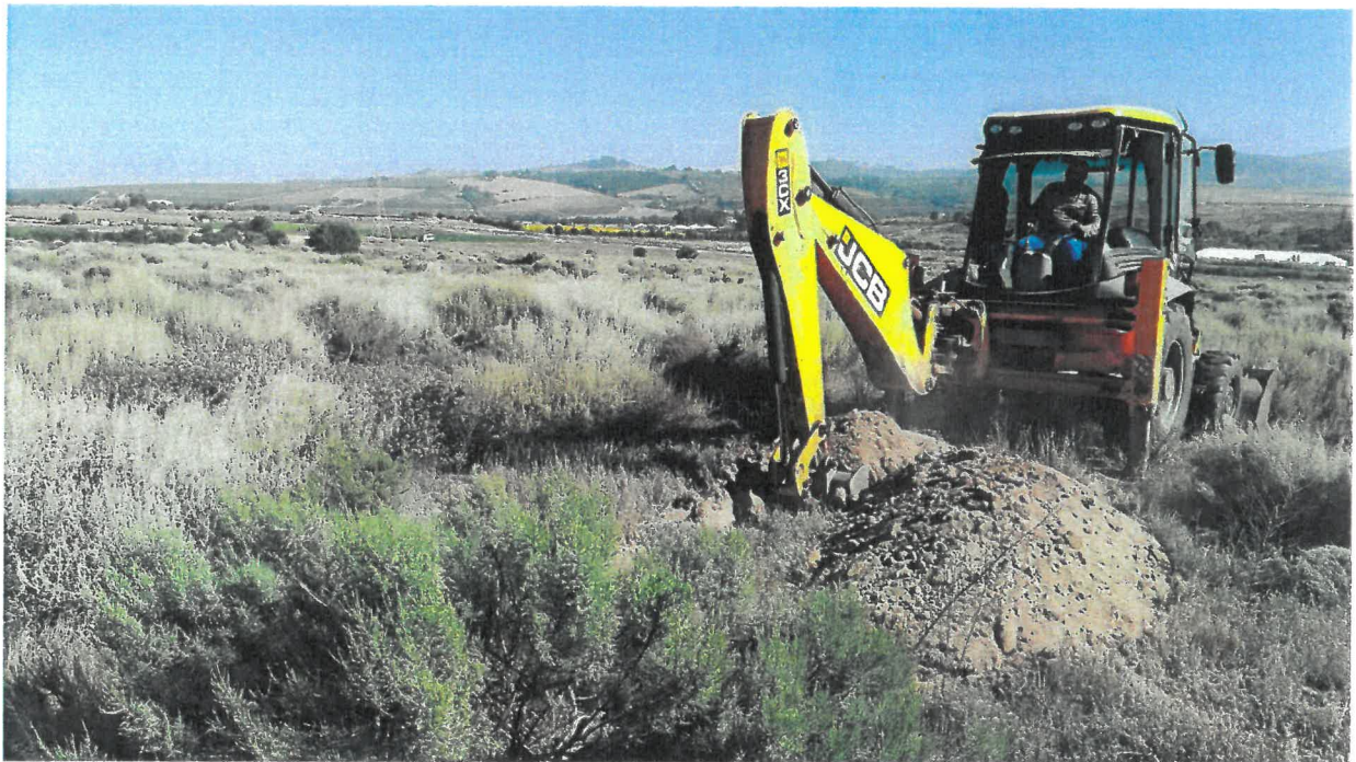
Figure 2. Site conditions looking down the focus area part of the site.
