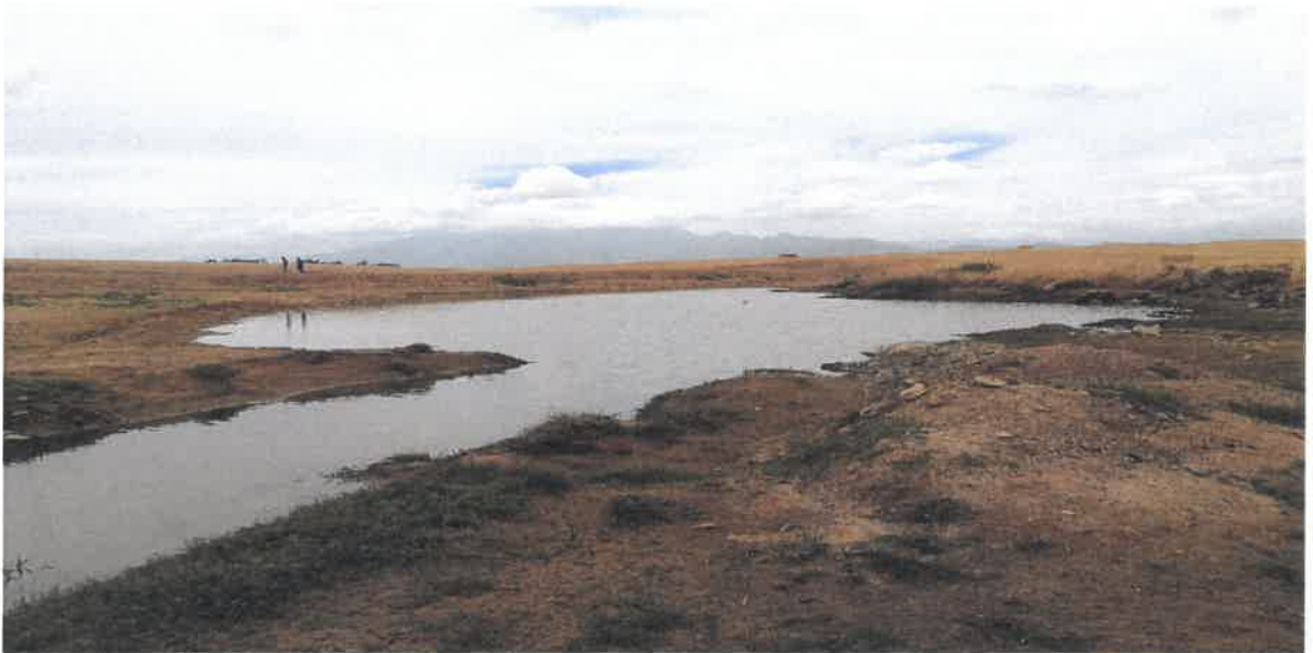
Photo 1: Construction of an in-stream dam on the Farm Rhenosterug No. 422, Riebeeek Kasteel
