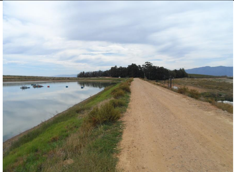
Figure 6: Standing on point B, on the dam wall, facing NE
