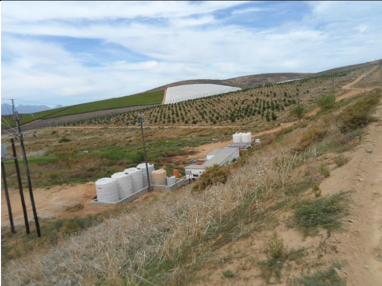
Figure 5: Standing on point B, on the dam wall, facing E to the existing pumphouse
