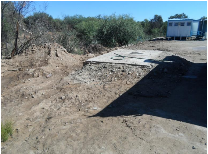
Photo 5: Conservancy tank near completed units (taken from position 2)
