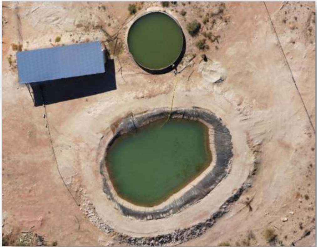
Photo 2: HDPE lined raw water storage dams
