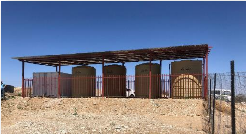
Photo 4: Water Treatment plant and 5 x 10 000 litre potable water storage tanks
