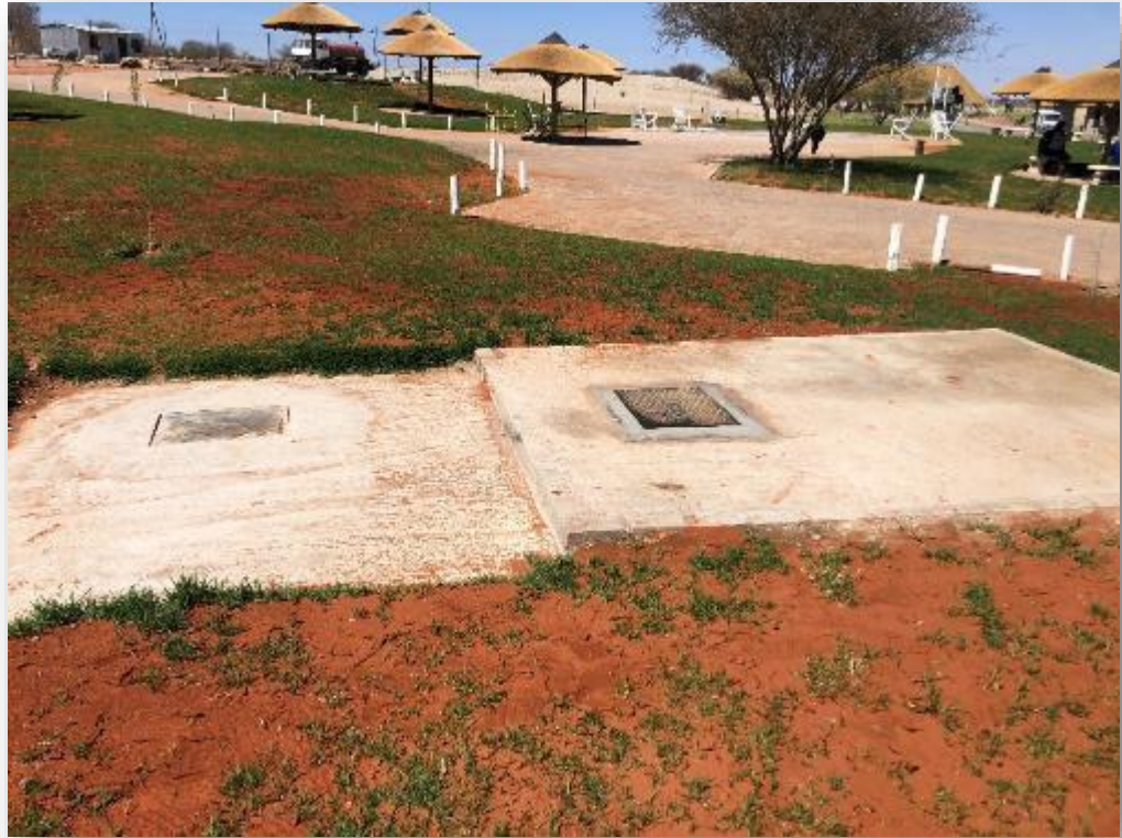
Photo 5: Sewer conservancy tank
