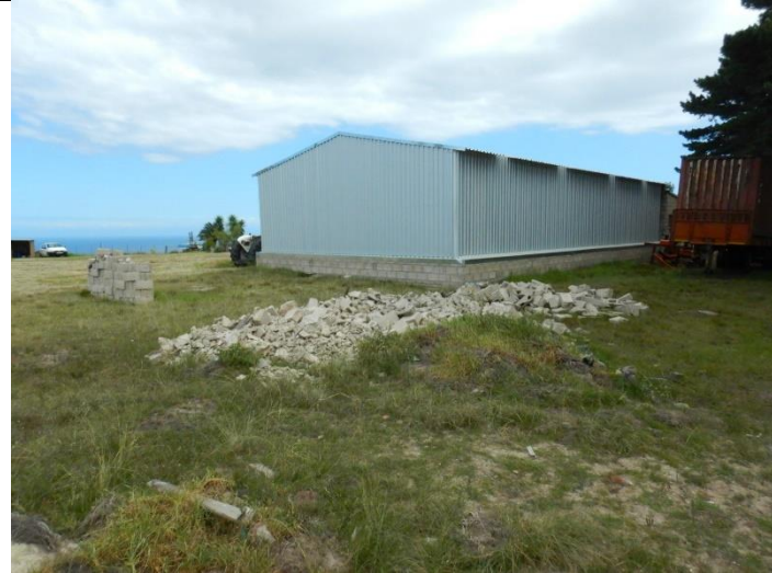
Figure 2: Photo taken on site facing South-West
