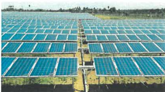
Figure 1: Single axis solar PV module tables raised 500mm above ground level (to a maximum tilt height of 3m). Proposed associated infrastructure includes a fenced construction staging area, a maintenance shed, inverter-transformer stations on concrete pads, office buildings and maintenance shed/s, a switch panel for connection to the power grid, all within the 218ha site.
