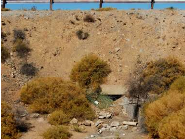
Figure 10 Another blocked culvert
