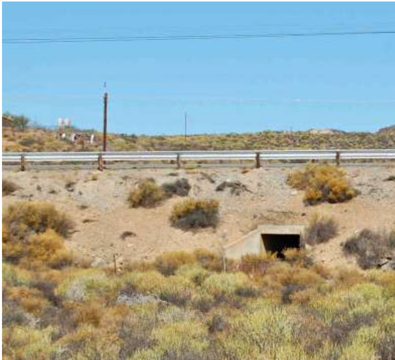
Figure 11 Box culvert
