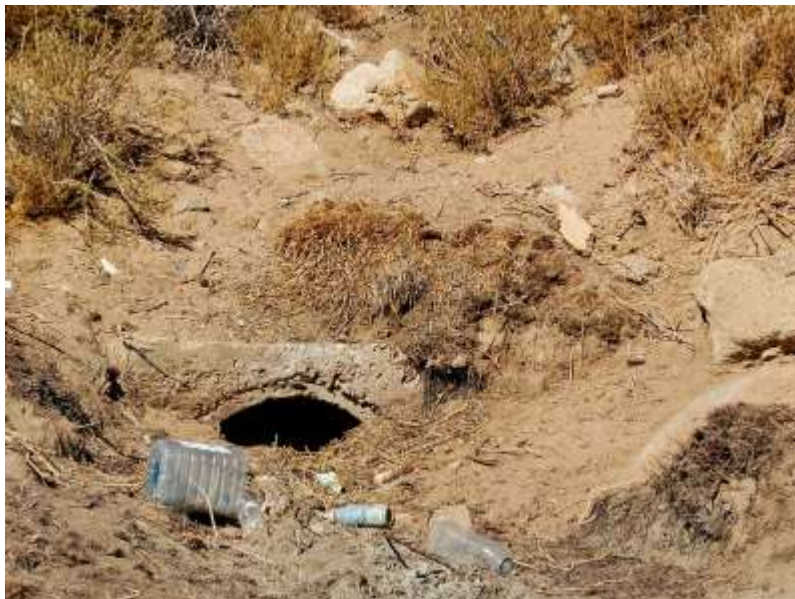
Figure 9 Blocked Culvert
